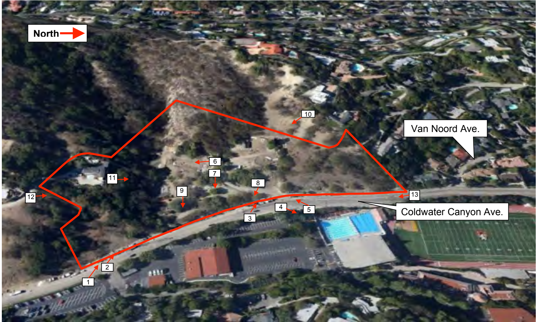
Figure 3.1-1 Aerial View of Development Site (location of proposed Parking Structure)
